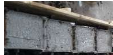
b. concreting samples
