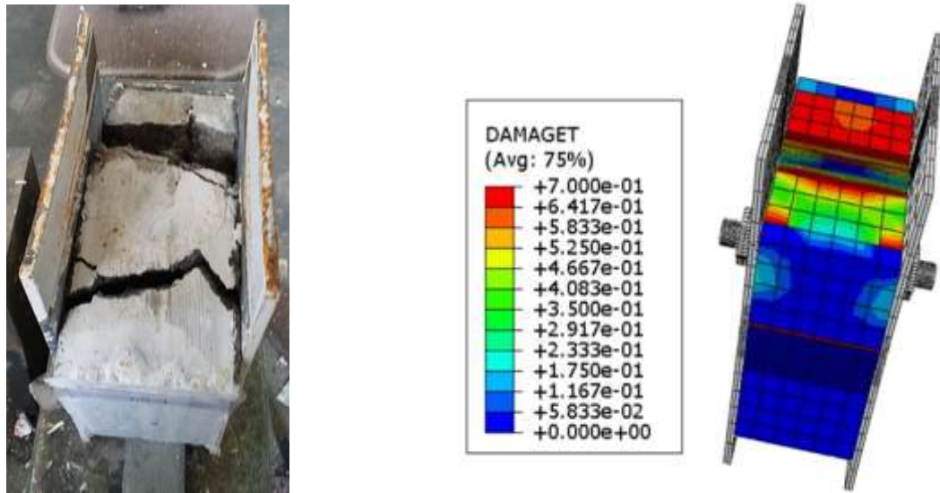
concrete cracking failure (sample 6S-4)
