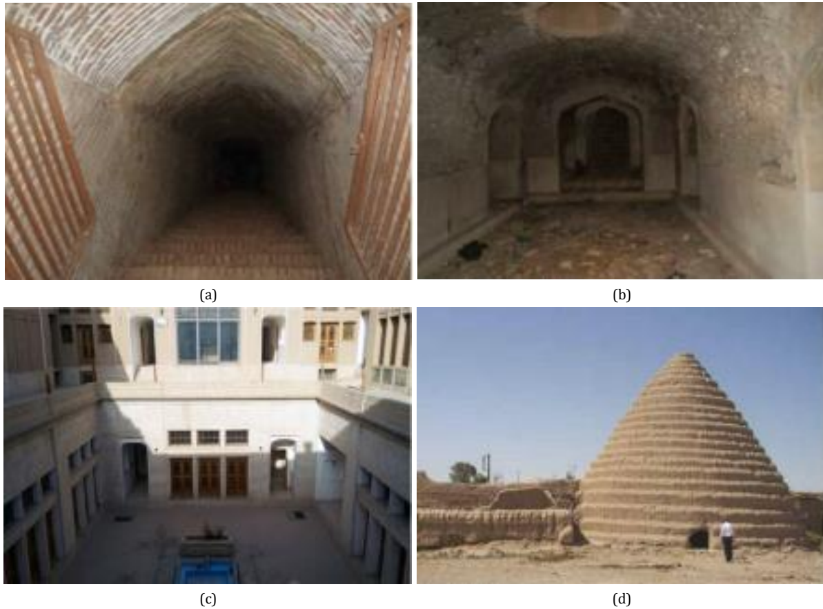
Figure 2. (a) Sardab (Cellar) [29]; (b) Shavadan [30]; (c) Sunken courtyard (Goudal Baghche) [31]; (d) ice-pit (yakhchal) [32].
