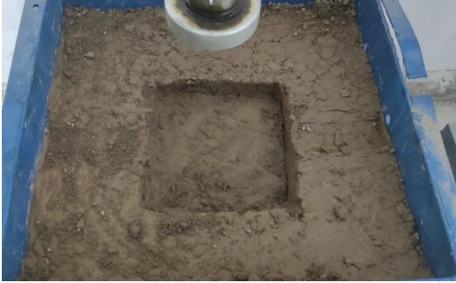
Fig. 12. Trench under the square footing.
