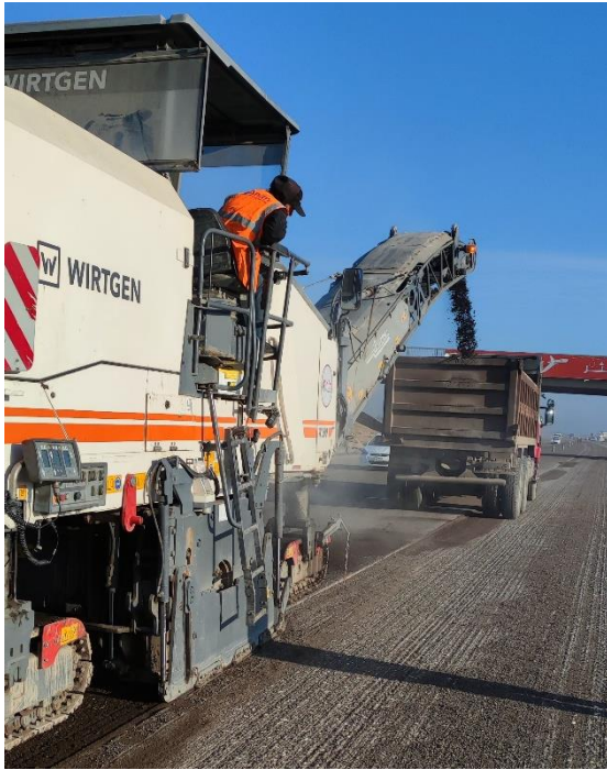
Fig. 1. Scraping up damaged asphalt, Baghdad – Babylon highway-Iraq (2021).
