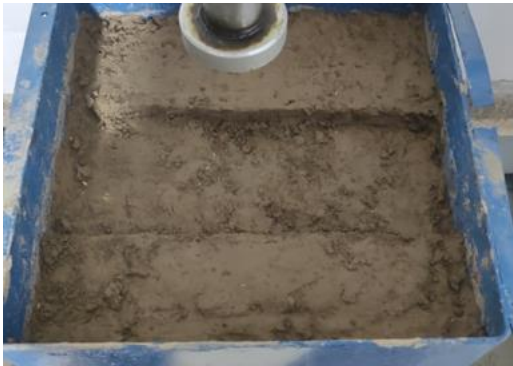
Fig. 14. Trench under the strip footing.
