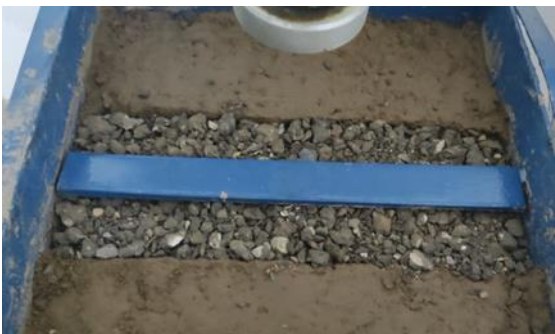
Fig. 15. RAP layer under the strip footing.
