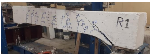
Fig. 7. Cracks pattern at failure for beam (R1).
