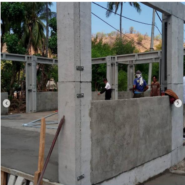
Fig. 5. Examples of RISHA Construction in the Field.
