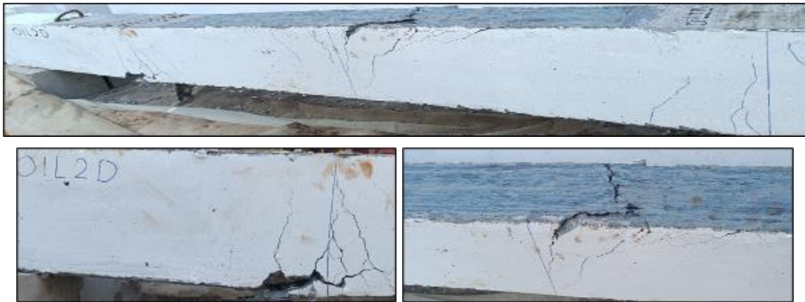
Fig. 14. Rupture of CFRP Failure Mode.
