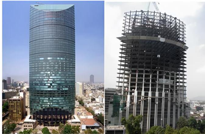
**Fig. 13.** Mega-brace dampers installed in the walls of Torre Mayor Tower during and after construction [3].
