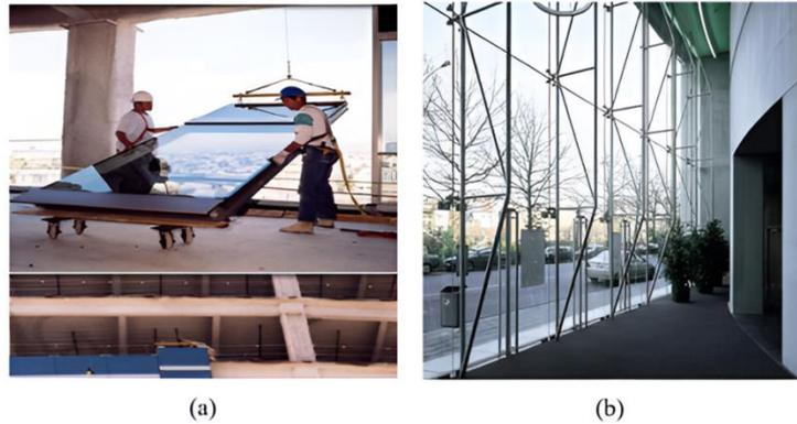
**Fig. 5.** (a) Construction process of curtain wall system; (b) implementation of bolted glazing façade system [35].
