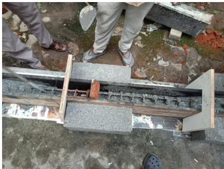
a) arranged reinforcement in the RC beam mould.
