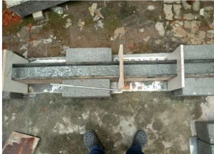
b) pouring of engineered mix into the mould.
