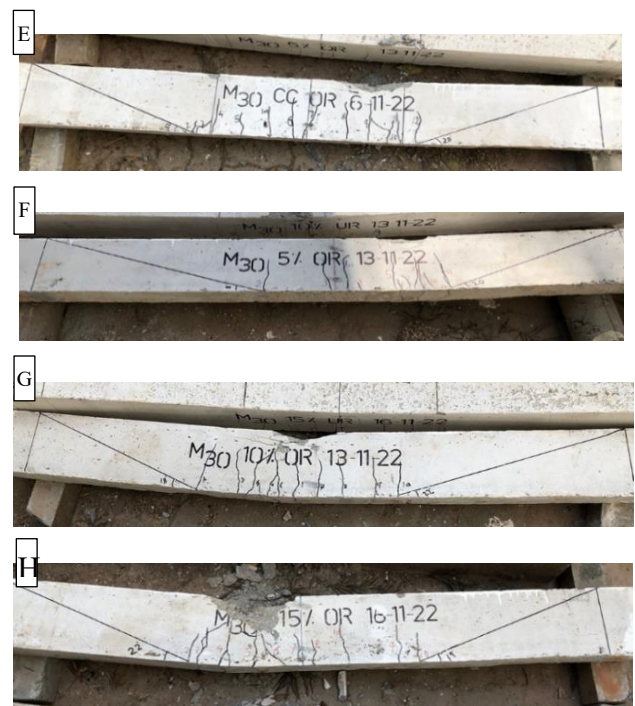
Fig. 7. The crack pattern of Alccofine-based M30 grade RCC beams for over-reinforced case.
