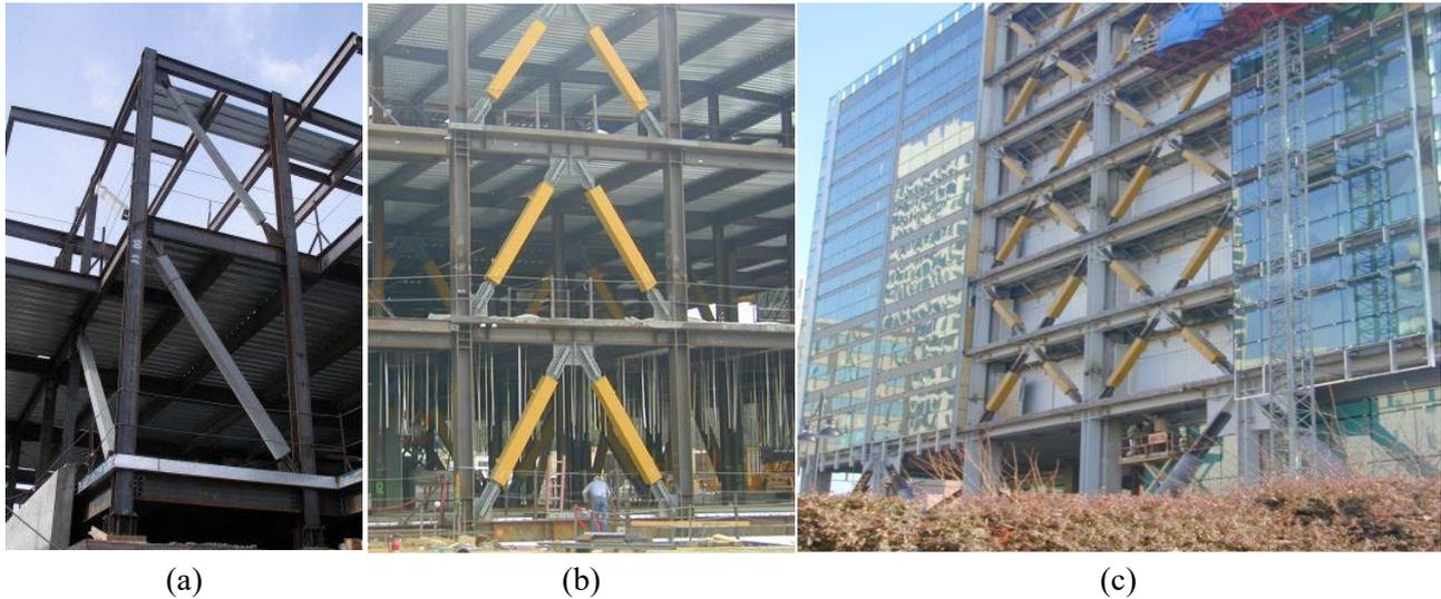
**Fig. 3.** Three different BRBs configurations: (a) single diagonal brace [28]; (b) inverted V-brace [29]; (c) X-brace [27].review of buckling restrained braces.
