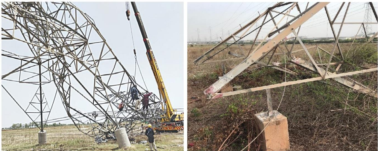
Fig. 1. Collapse of steel lattice tower due to wind load (Sindh, April 2022).
