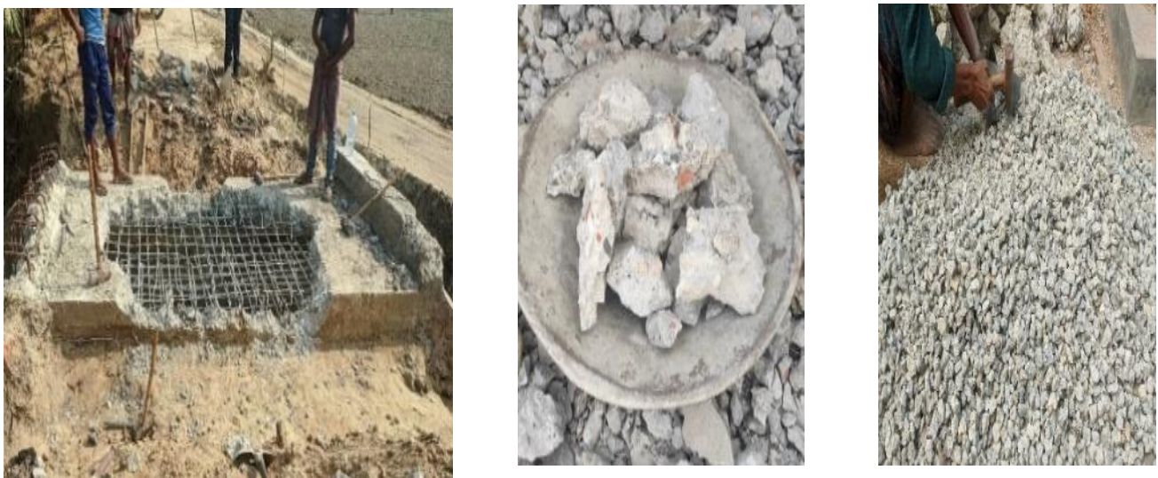
Fig. 1. Processing of recycled aggregate from demolished concrete.
