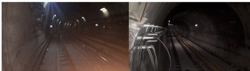
Figure 2: View of tunnel in Tehran subway
