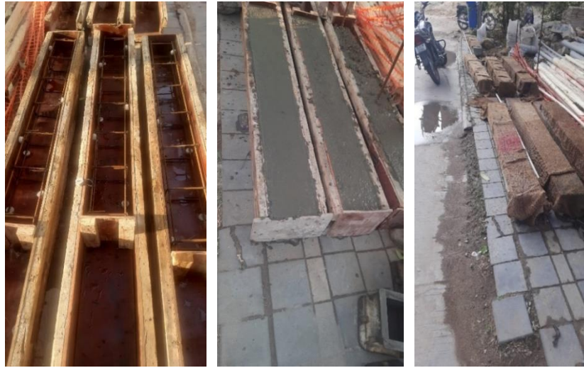
Fig. 2. Casting of Beams.
