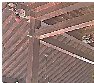
(a) Beam-to-main column joint.
