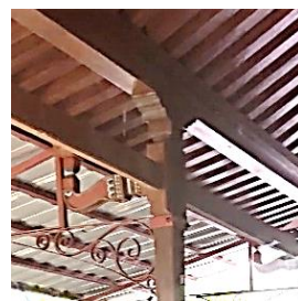
(b) beam-to-side column joint.
