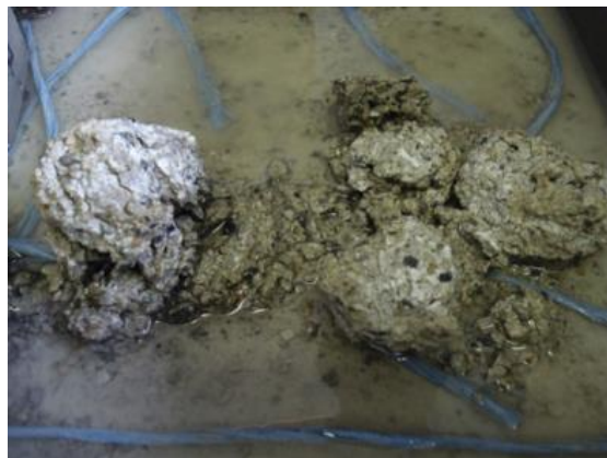
(b) The appearance of concrete under thaumasite sulfate attack
