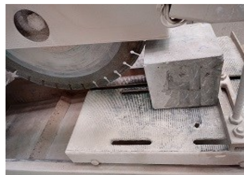
Fig. 2. Cutting the substrate concrete
