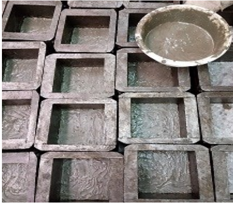
Fig. 3. Applying the grout and the repair layer over the concrete substrate
