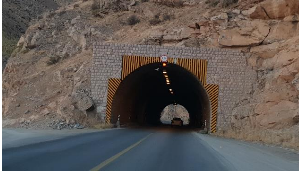
Fig. 2. View of entrance to third tunnel.
